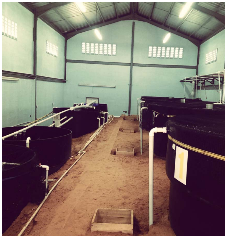
Figure 3 Phase 1 of the Tilapia Production Facility with a hatchery and grow out ponds
